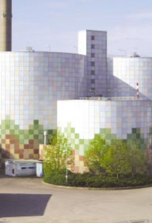
Digestion chambers at a sewage plant. Heated tanks, that contain several thousands cubic metres of sewage, are concealed under the tiles.
