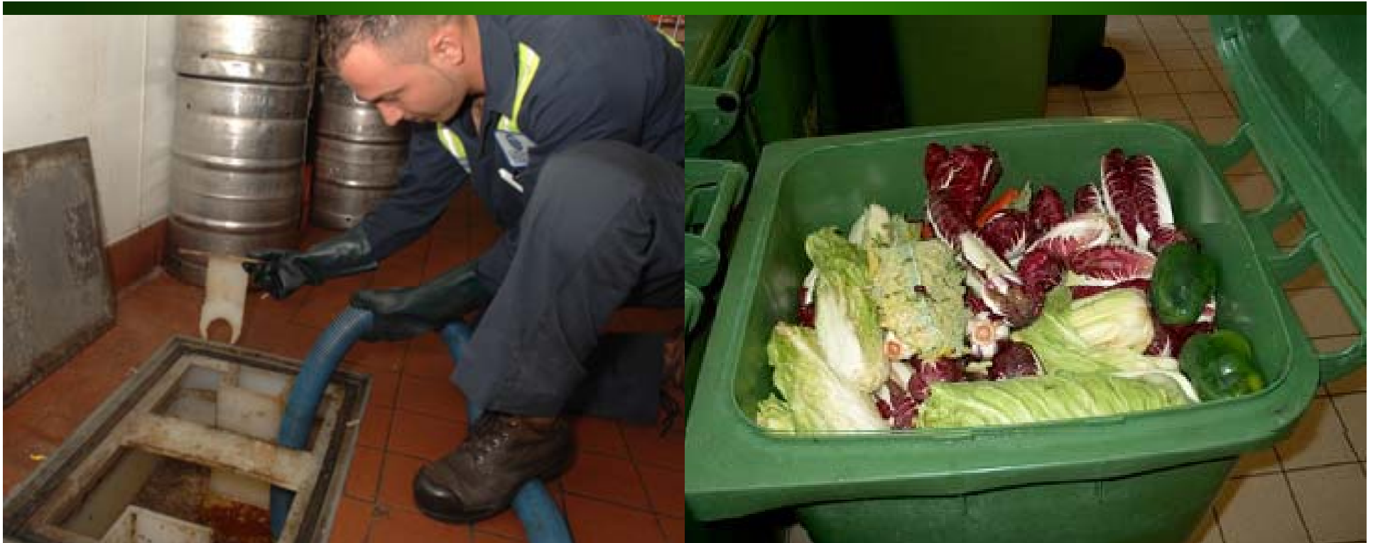
Fats, Oils, Grease
